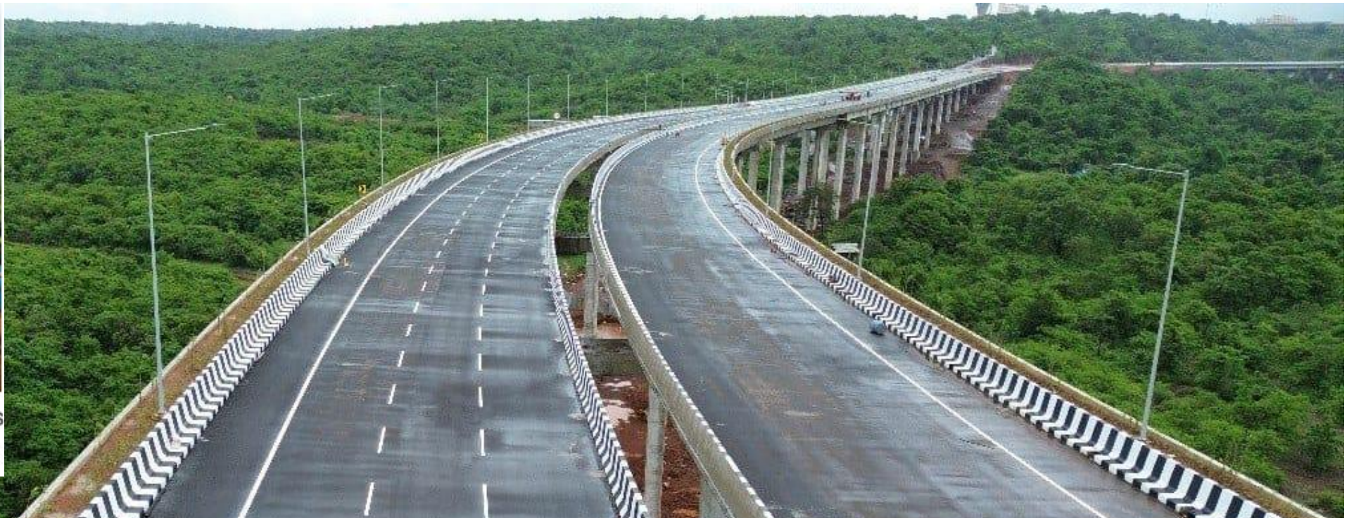
The elevated corridor consists of numerous piers that reach height of up to 40 meters.
